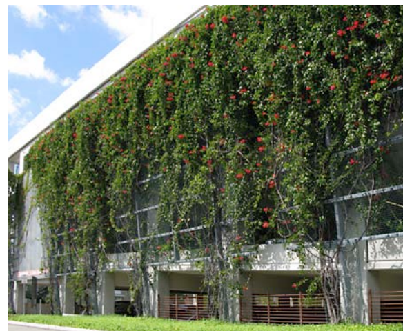
These vines planted directly into the ground have ample soil volume and correct spacing for full coverage to four stories, Fullerton, CA
