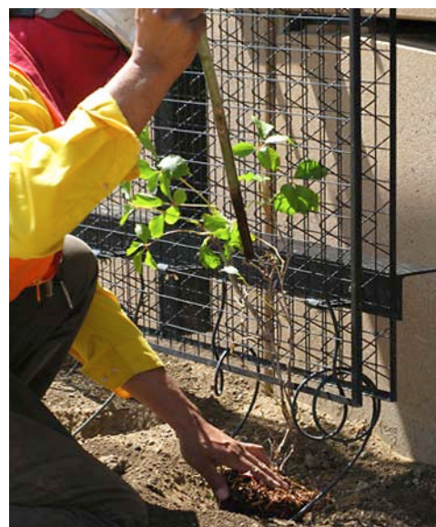
Proper soil preparation and plant spacing, with irrigation placed in advance, before mulch layer application
