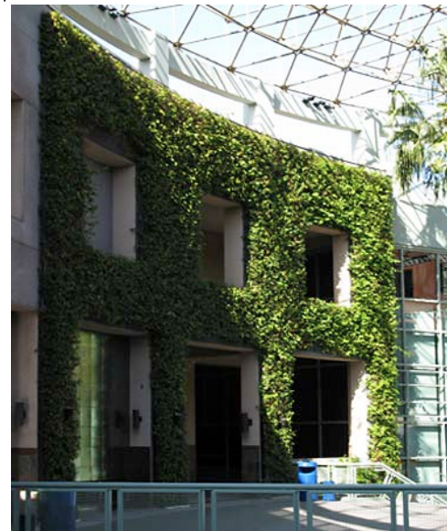
Proper soil volume, irrigation delivery and maintenance are successfully demonstrated in this 18 year old green facade installation, Universal City, CA
