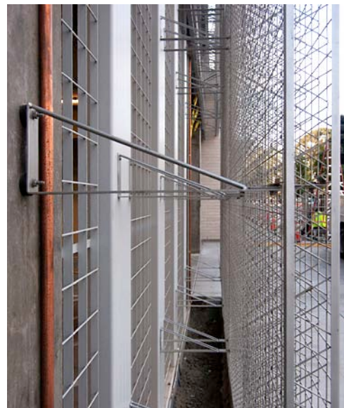
Wall mounted, modular three-dimensional panels, with standoff brackets, provide access to keep plants off the wall, Oakland, CA
